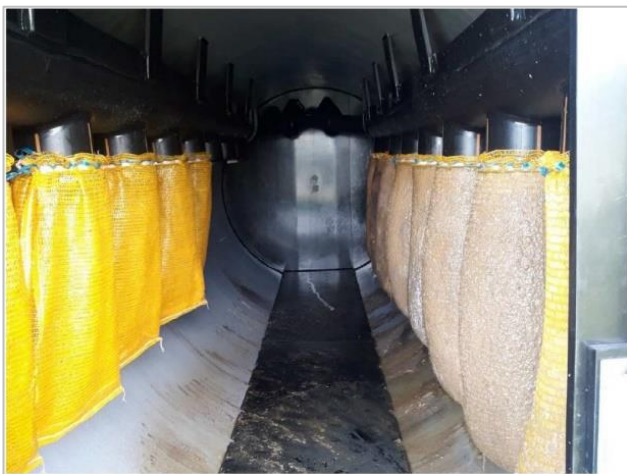
Filter bag plant Ostpreußen Hut
